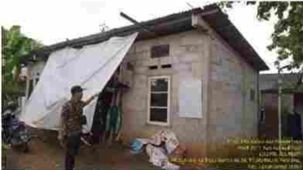
PHOTO BEFORE (DRI)
