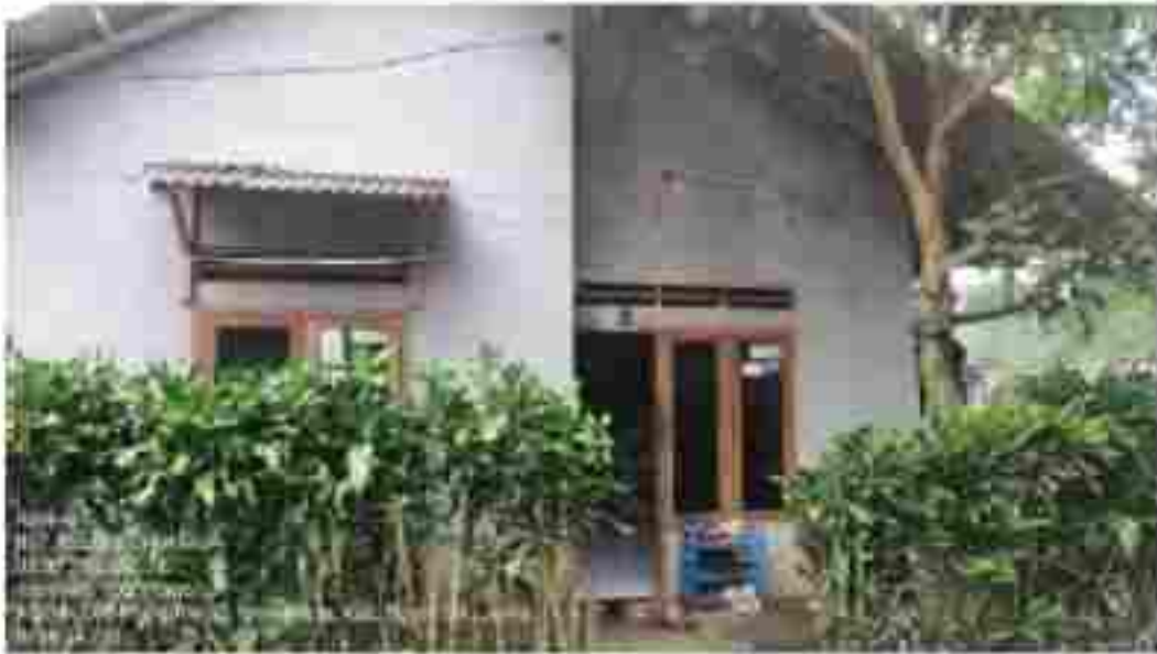
PHOTO BEFORE (DPR)
